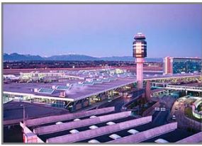
VANCOUVER EC Vanc. International Airport Asbestos Abatement $10M
